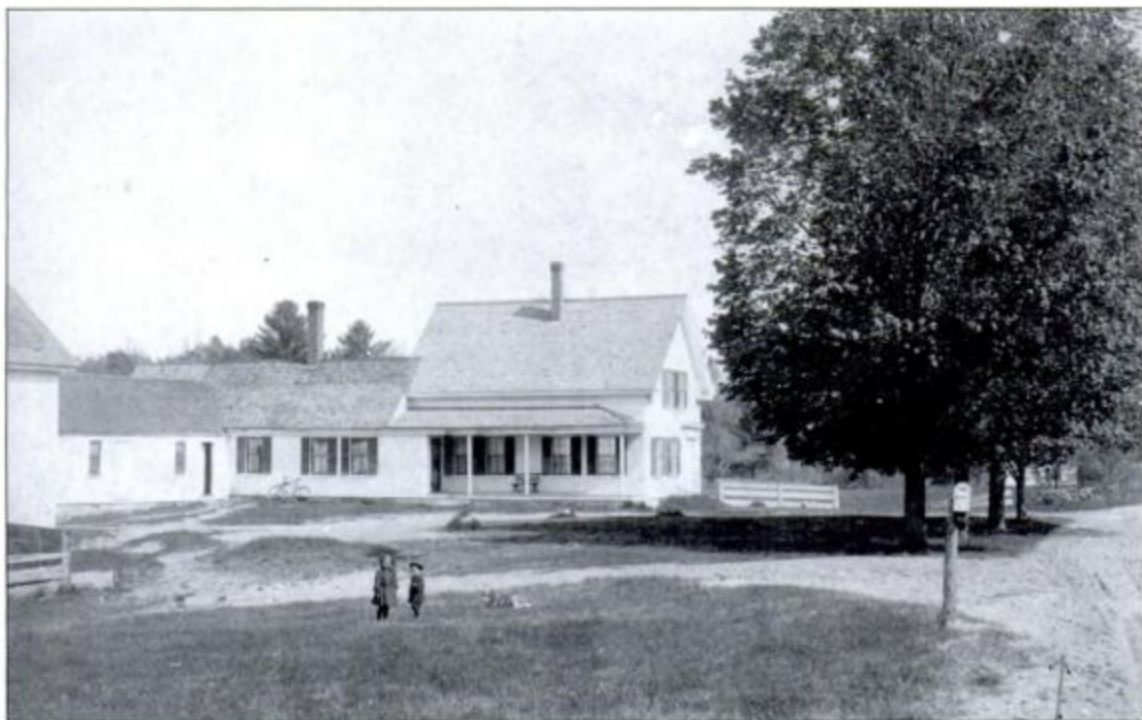
GILE HOME. Built in 1850 on 50 acres, the old Martin Gile home is located on Old Batchelder Road (today 5 Gile Road). The Gile school building can be seen under the tree at the right of this view on its original site. At one point, this was Joseph Mandile's poultry farm. It was also James and Blanche Clement's poultry farm from the 1930s to mid-1940s. This was just one of many chicken farms in Raymond at the time. (Courtesy of the Raymond Historical Society.)
